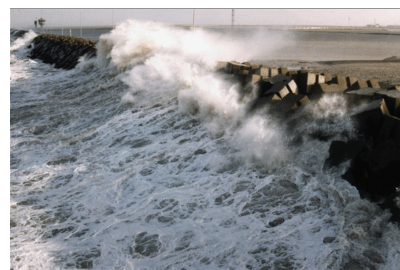
Waves attacking a rubble mound breakwater (Zeebrugge harbour, Belgium)
