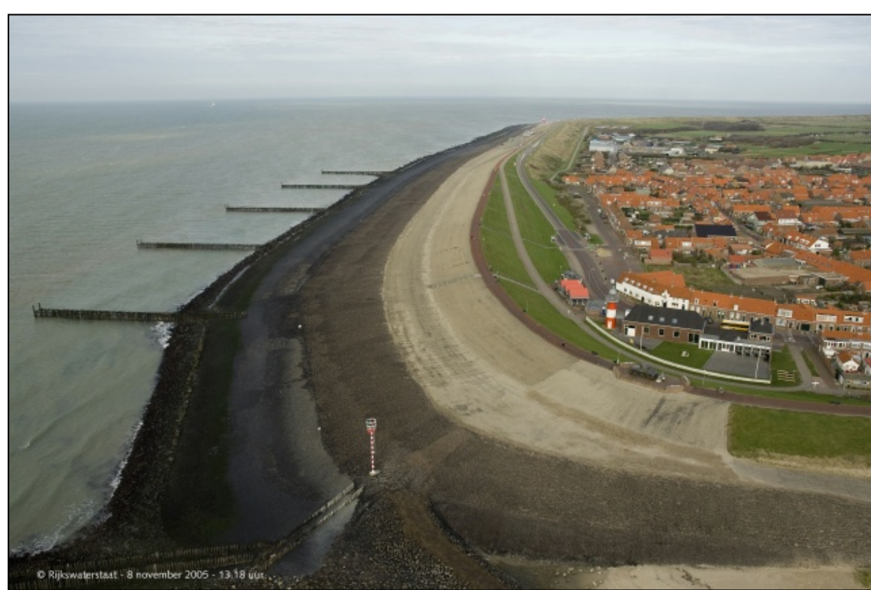
Seadike: groynes, berm, maintenance path, revetment and grass cover (Westkapelle, The Netherlands)
