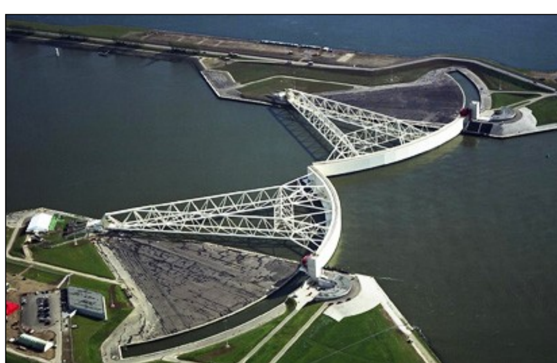
Delta Works: Maeslantkering storm-surge barrier (Rotterdam, The Netherlands)
