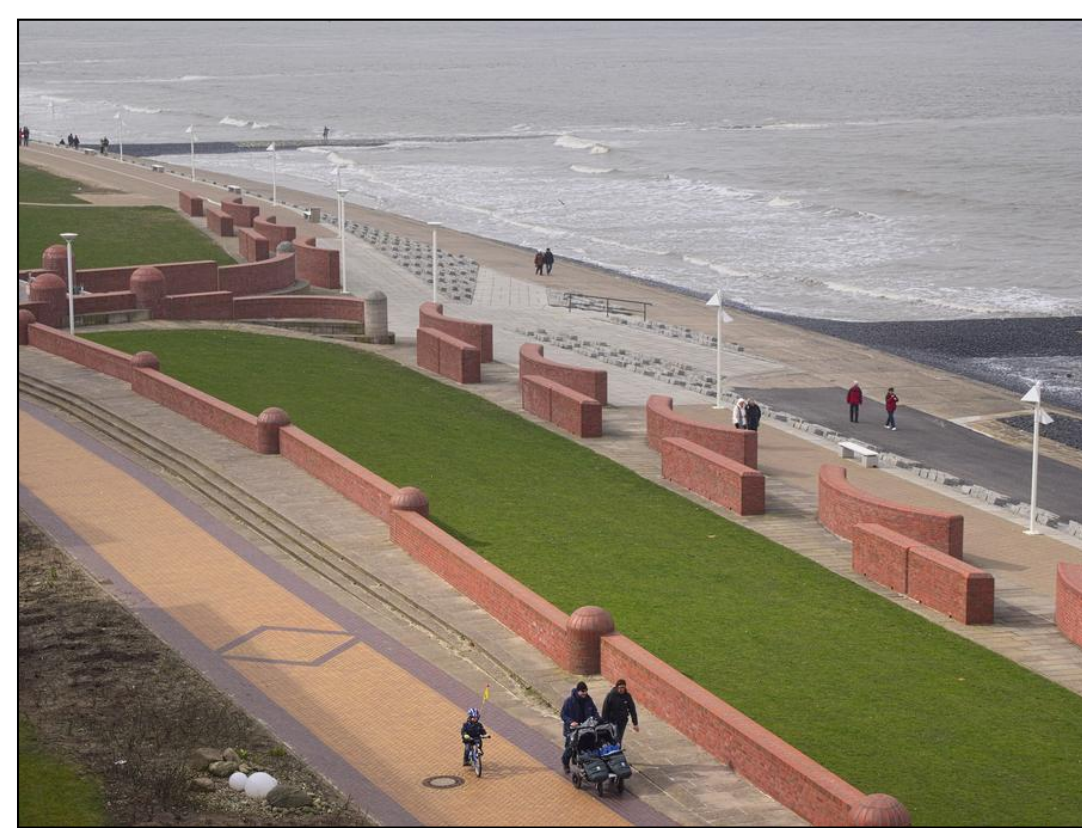
Dike with concrete revetment and storm wall elements (Norderney, Germany)
