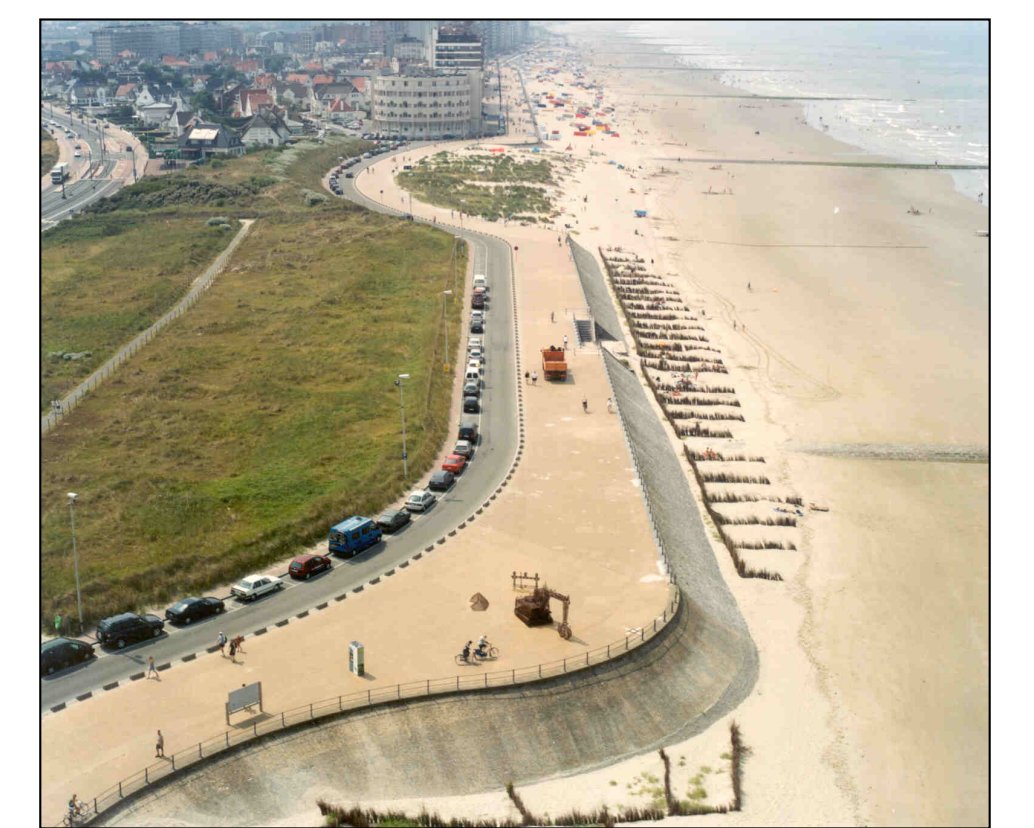
Combined dike and dune system (Westende, Belgium) Source: afdeling KUST
