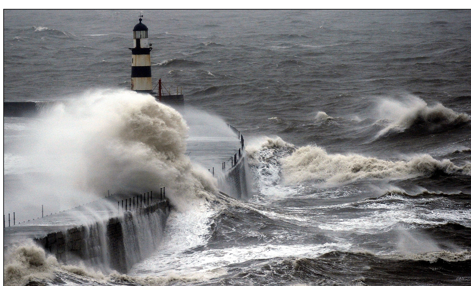
Seawall to block the waves (Seaham, UK)
