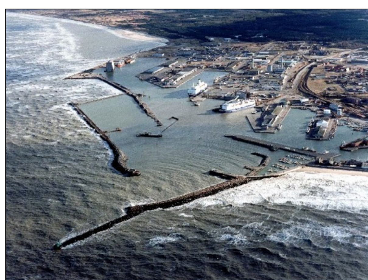
Harbour with quay wall and rubble mound breakwater (Hirtshals, Denmark)
